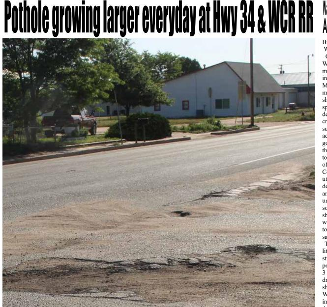
The pothole at the intersection of Hwy 34 and RR is growing larger everyday. Semi's are having to make wide turns to avoid the pothole. CDOT plans on working on the pothole sometime this week. Photo by Jerry Patterson.
